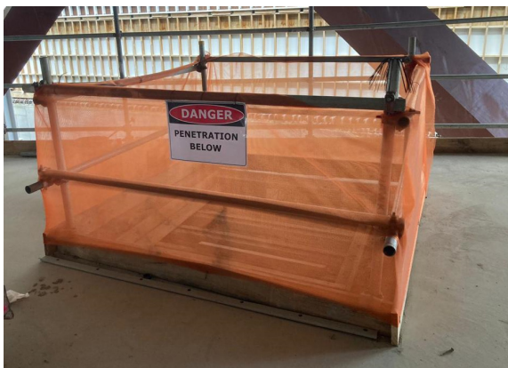
Penetration protection and signage.
